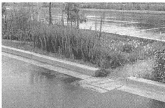
FIGURE 5-17 Bioretention during a storm event at the University of Maryland.
