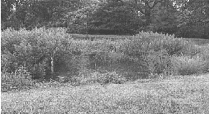
FIGURE 5-19 Retrofit bioinfiltration at Villanova University immediately following a storm event.
